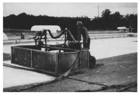
FIGURE 12.6 Robotic sprayer applying polyurethane foam.
