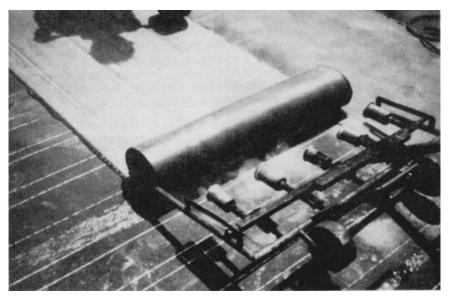
FIGURE 12.4 Torch application of atactic polypropylene (APP) modified bitumen membrane.
